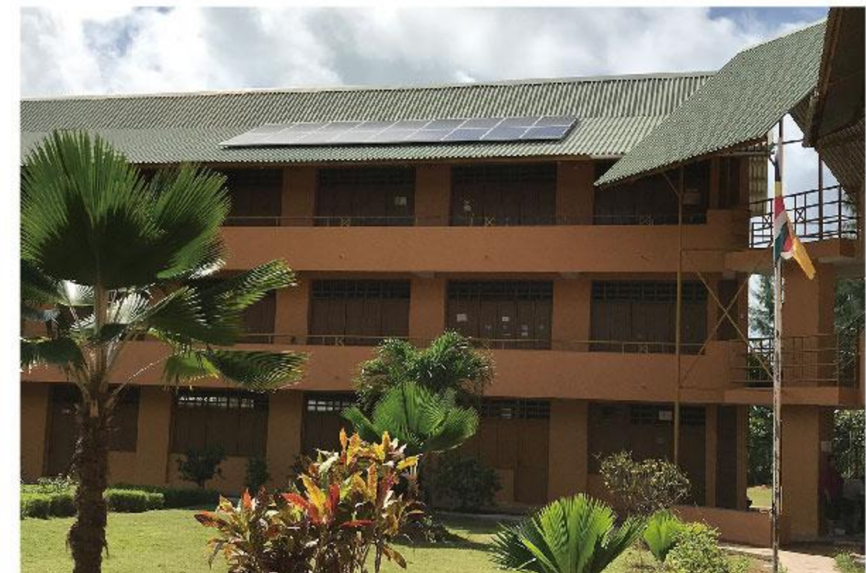
China and Seychelles jointly build a low-carbon demonstration zone project
